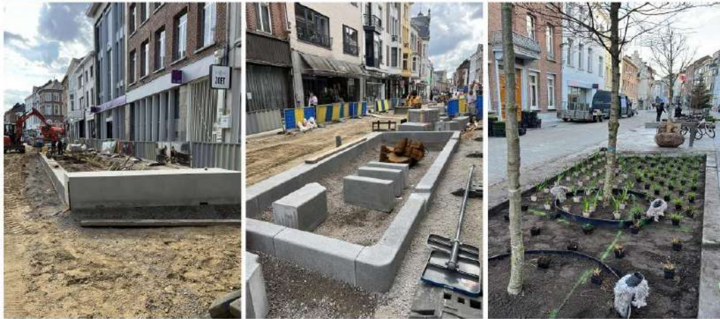
Construction progress (top) and the almost finished street (bottom).
